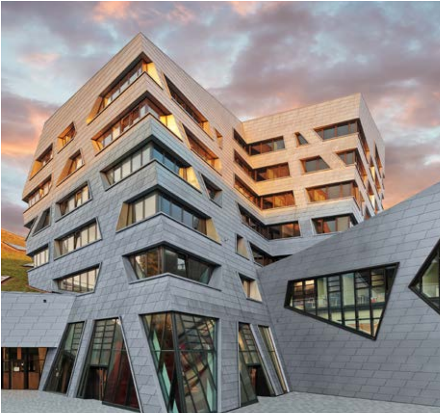
Central Building of the Leuphana University, Luneburg, Germany
