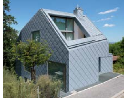
Split-Level, Stuttgart, Germany
