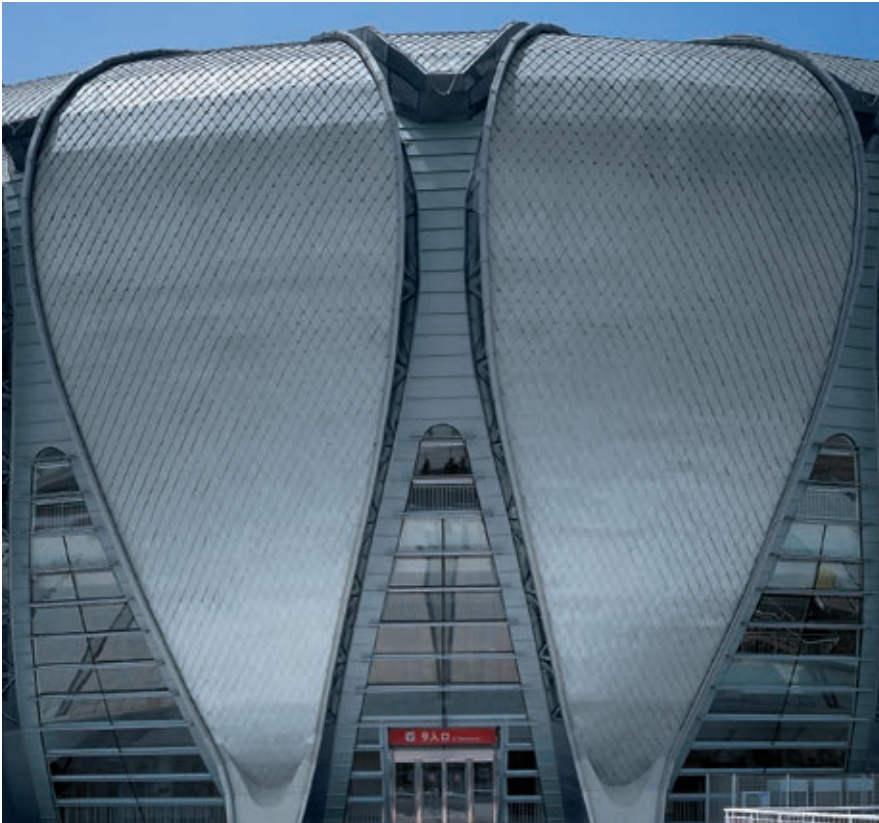
Olympic Stadium, Jinan, China
