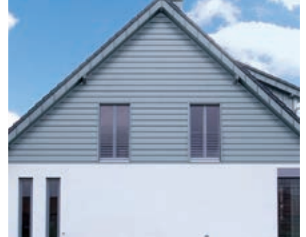
Gable cladding at residential building
