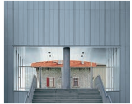
Telecom Giubiasco, Giubiasco, Switzerland
